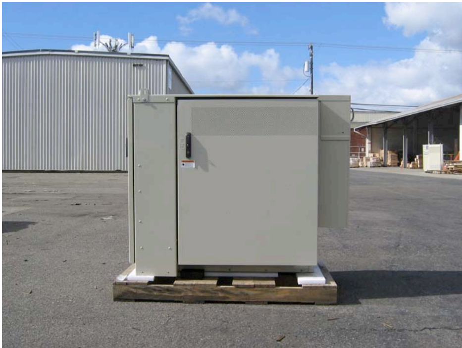
Typical utility box installation for Project Lightspeed
